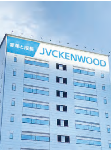
Head Office & Yokohama Business Center
